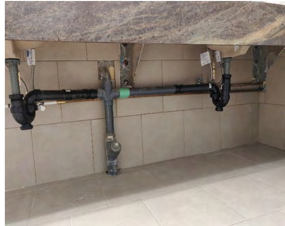
Figure 5-4 Washroom Lavatory Plumbing
