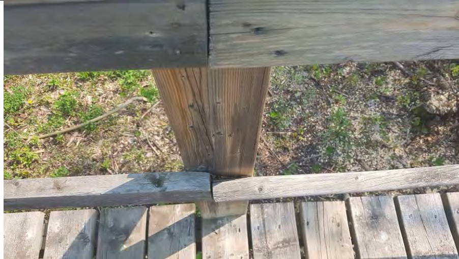
Photo 10 View of warping rail and loose connections
