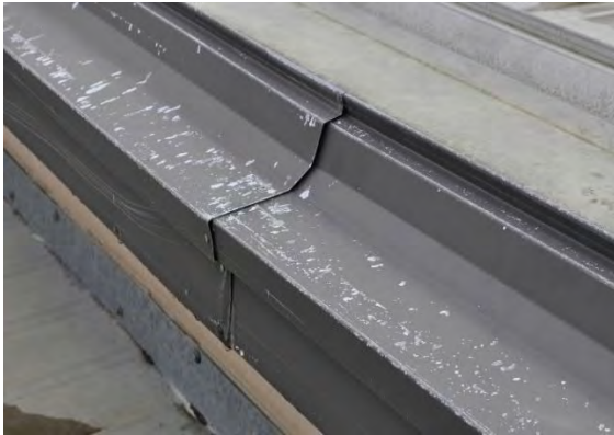
Figure 3-35 Flashing Joint/Deteriorating Finish
