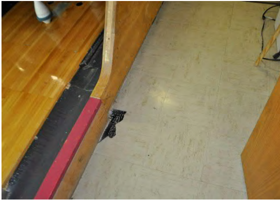
Figure 3-59 Service Aisle Entrance Damaged Tile
