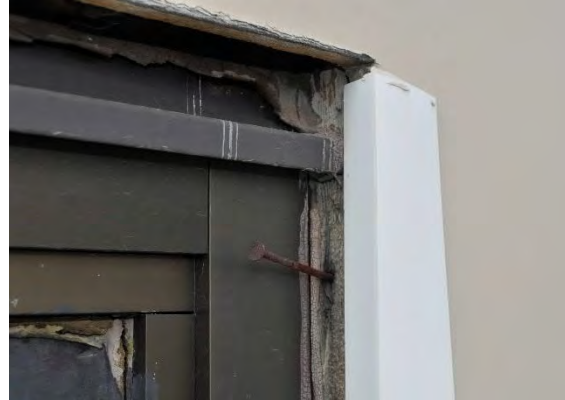
Figure 3-28 Clerestory Window Flashings, Sealants and Cracking & Peeling Coating Over Glazing
