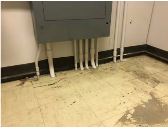
Figure 4-5 Viewing Settlement Along Wall in Electrical Room
