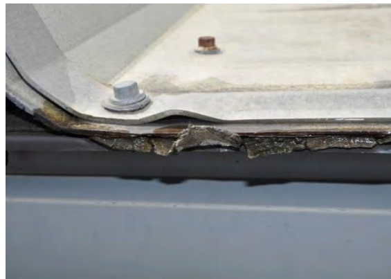
Figure 3-42 Deteriorated Gasket Material
