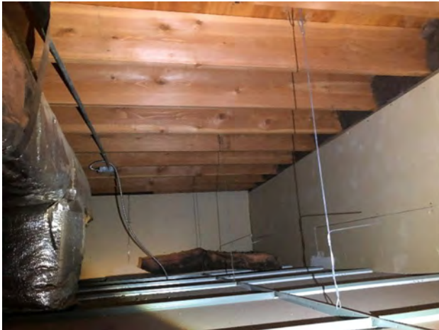
Figure 4-16 Viewing the Typical Condition of Timber Roofing
