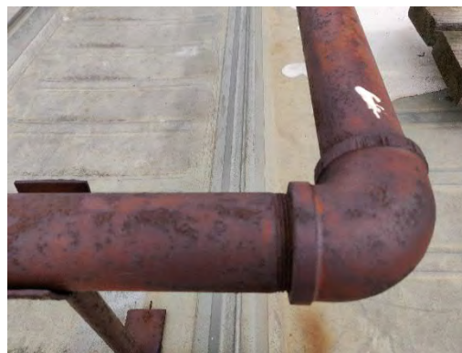
Figure 5-13 Surface Corrosion of Gas Piping
