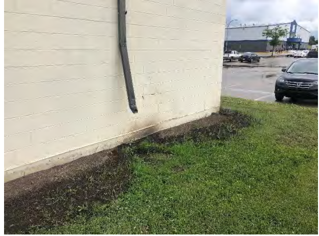
Figure 2-7 Example of Cut Downspout Without Splash Pad
