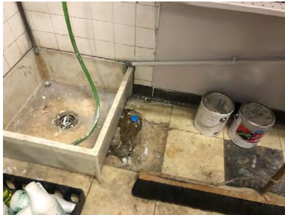
Figure 4-7 Area Requiring Concrete Patching in Janitor's Room
