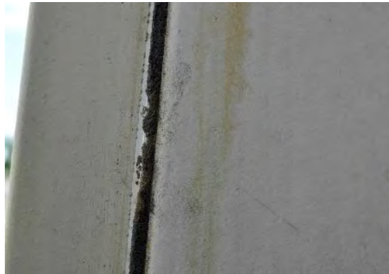
Figure 3-21 Deteriorated Weather-stripping
