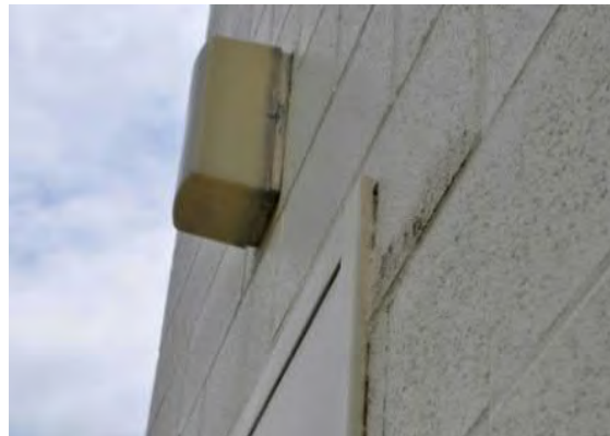
Figure 3-17 Gap Between Frame and Masonry Block Wall
