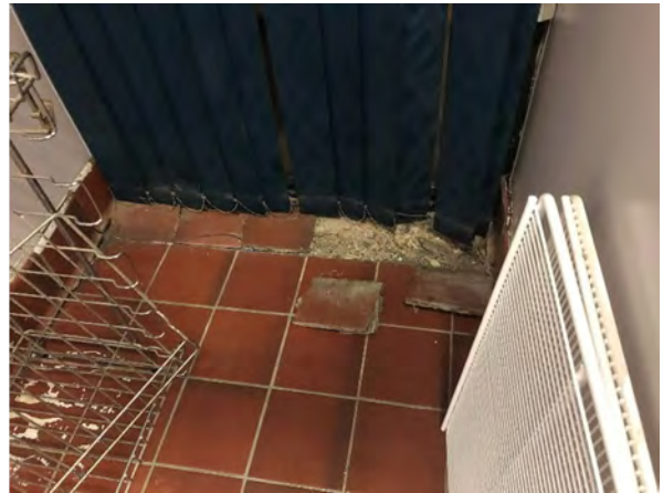
Figure 4-4 Substantial Settlement Near the Foundation Joint of the Window of the Snack Bar
