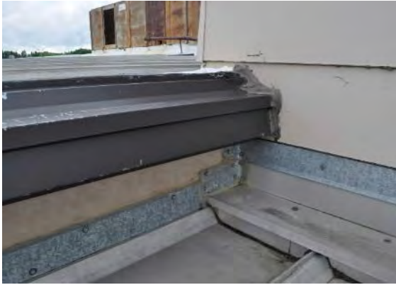
Figure 3-39 North Clerestory Wall Sealant
