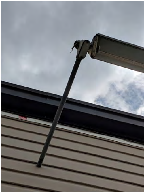
Figure 6-14 Abandoned Conduit and Exposed Wiring (West Side)
