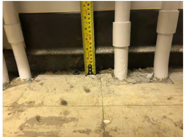
Figure 4-6 Approximately 60 mm of Settlement in Electrical Room
