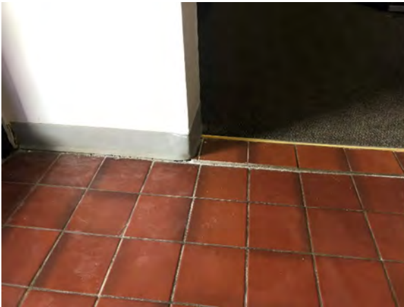
Figure 4-3 Slight Settle in the Tiled Surface Near the Main Entrance and in the Storage Room
