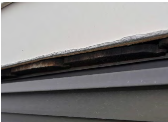
Figure 3-25 Clerestory Windows No Head Flashing
