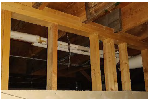
Figure 5-2 Insulation on New Domestic Water Piping
