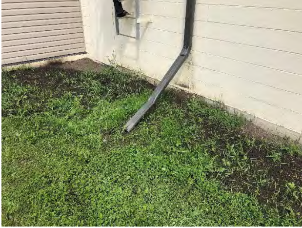
Figure 2-6 Example of Damaged Downspout Without Splash Pad
