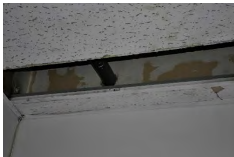
Figure 3-68 Mech Room Pipe (Not Fire Sealed)
