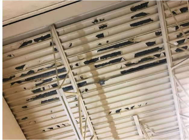
Figure 4-13 Viewing Flaking Paint of Roof Decking Above Pin Equipment
