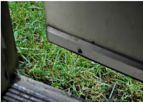
Figure 3-16 No Landing Apron, Deteriorated Door Sweep
