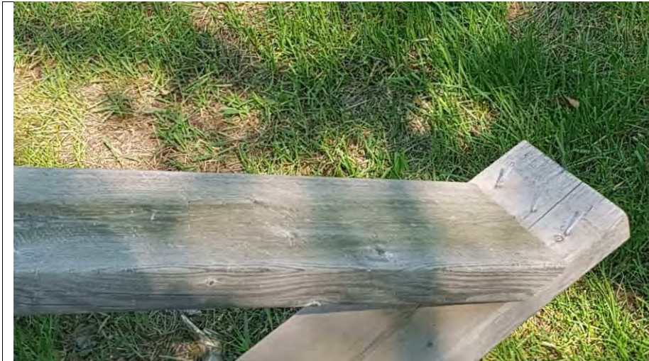
Photo 7 View of vertical rail brace no longer nailed
