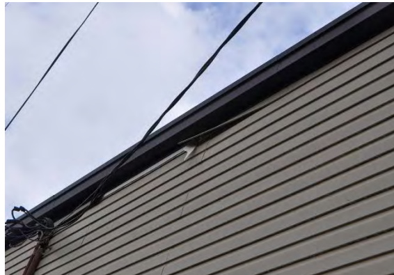
Figure 3-4 Damaged Vinyl Siding
