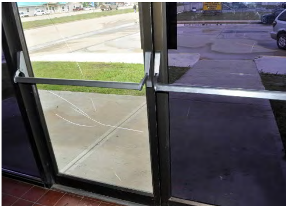
Figure 3-12 Main Entrance – Cracked Glazing
