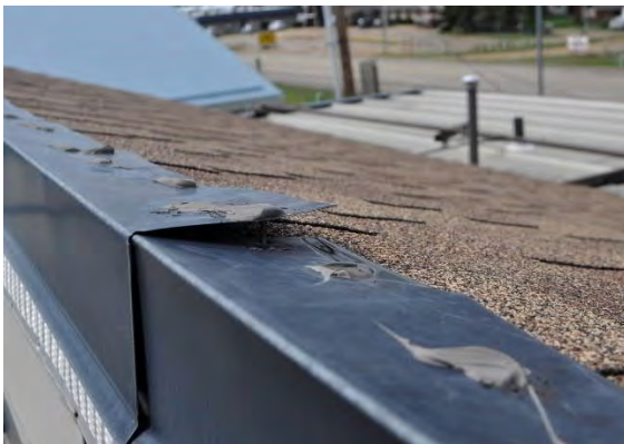
Figure 3-37 Flashing Joint/Pulled Fasteners
