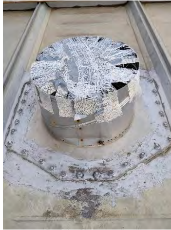
Figure 5-21 Missing Roof Vent
