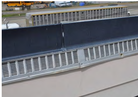
Figure 3-38 Clerestory Roof Vents
