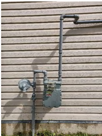
Figure 5-11 Gas Meter Installation
