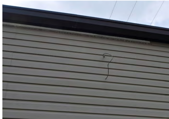
Figure 3-6 Missing Vinyl Siding Unsealed Cable Penetration
