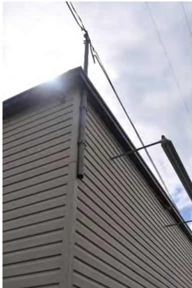
Figure 3-7 Electrical Mast Through Gutter
