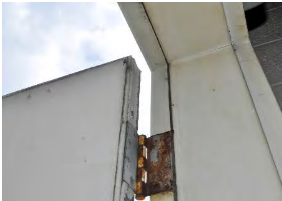
Figure 3-20 Rusted Hardware
