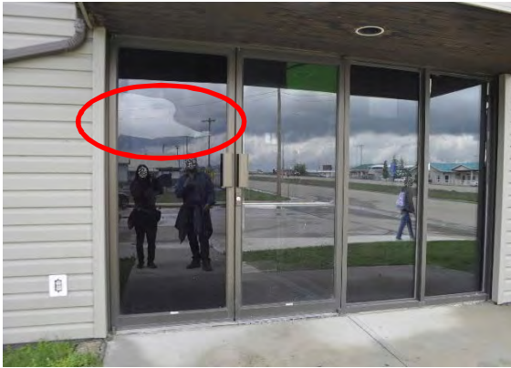
Figure 3-10 Main Entrance – Peel & Stick Tinting
