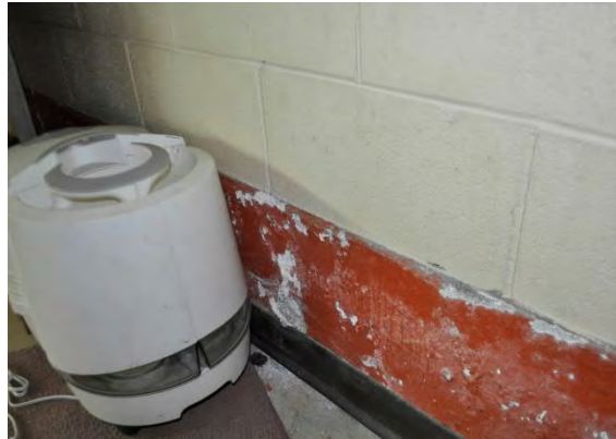
Figure 3-46 Moisture Damage
