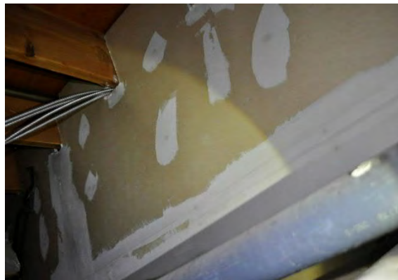
Figure 3-66 Armoured Cabling Not Fire Sealed
