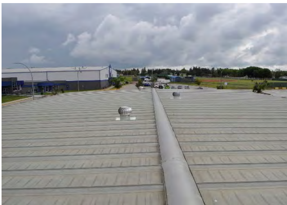
Figure 3-33 Low Slope Metal Roofing System
