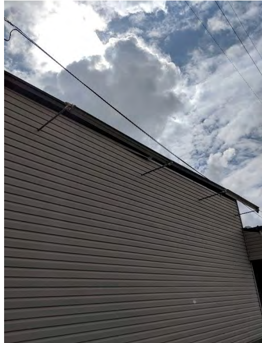
Figure 6-15 Abandoned Conduit (West Side)
