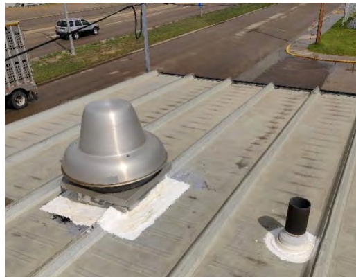
Figure 5-18 Washroom Exhaust Fan
