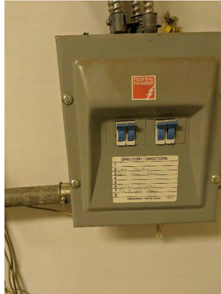
Figure 6-6 8cct Sub Panel
