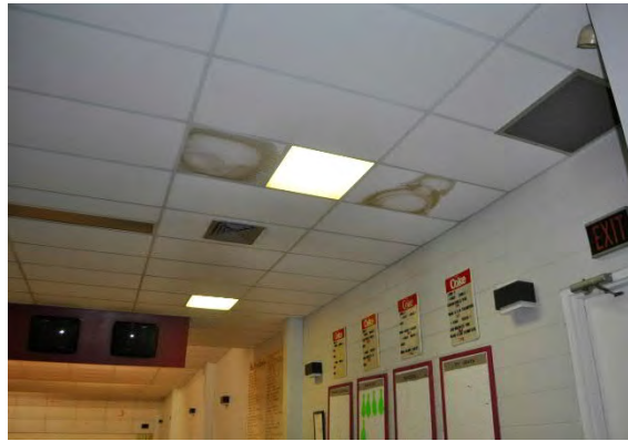
Figure 3-64 Stained Ceiling Tiles
