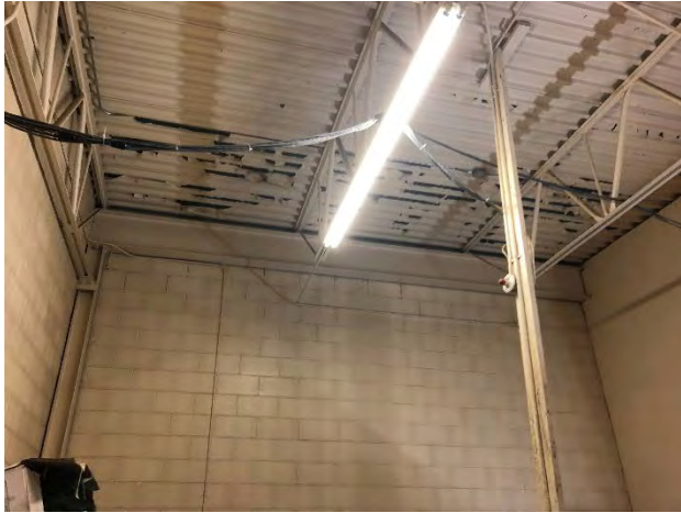
Figure 4-12 Viewing Flaking Paint of Roof Decking Above Pin Equipment
