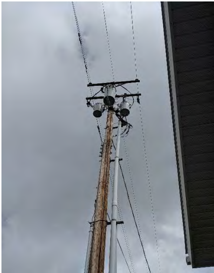
Figure 6-1 Utility Pole Mounted Transformer
