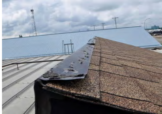
Figure 3-36 Clerestory Roof Peak Flashings
