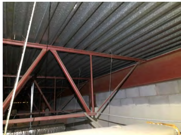
Figure 4-15 Viewing Steel Pick Up Beam at South Wall of Bowling Lanes
