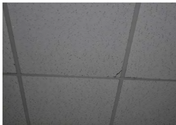
Figure 3-62 Broken Tile
