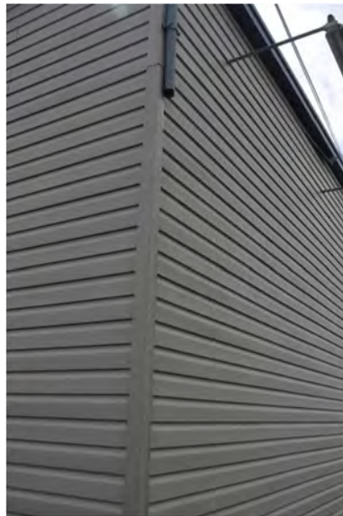
Figure 3-8 Stained Siding & Unsealed Penetrations
