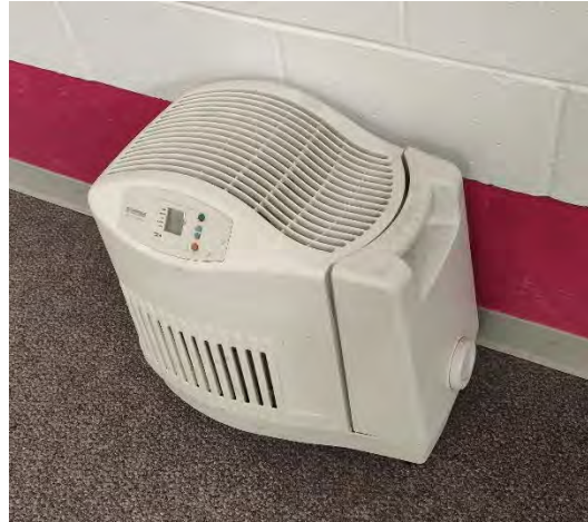
Figure 5-17 Portable Humidifiers in Bowling Area
