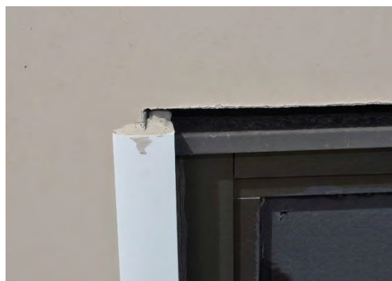
Figure 3-26 Clerestory Window Side Flashing and Sealant
