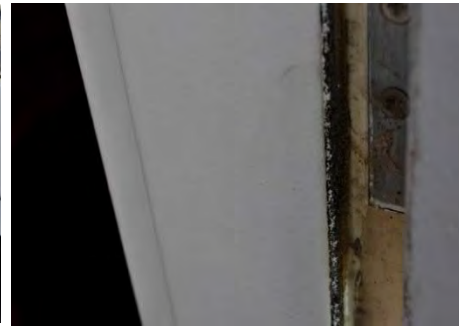
Figure 3-24 Weather-stripping
