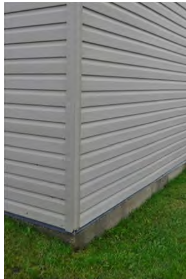
Figure 3-9 Damaged Siding Corner Trim
