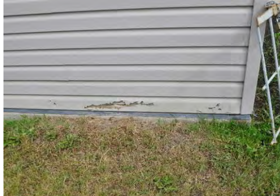
Figure 3-2 Damaged Vinyl Siding
