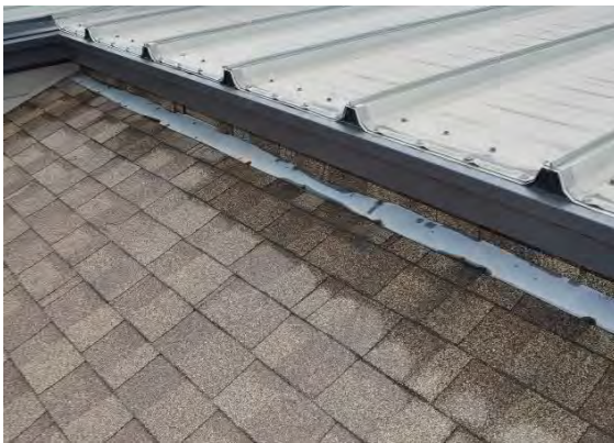
Figure 3-41 North Entrance Roof Rusted Flashing
