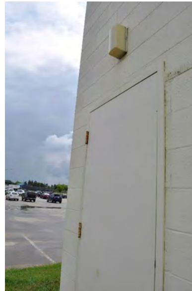
Figure 3-15 Northeast Exit Door No Head Flashing
