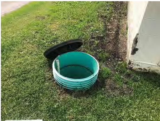
Figure 2-4 Viewing Buried Drainage Sump and Lid
