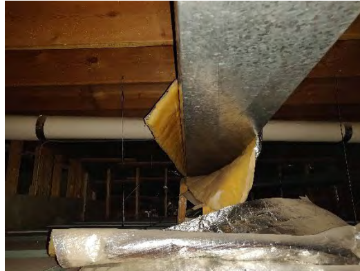
Figure 5-19 Typical Duct Insulation in Ceiling
