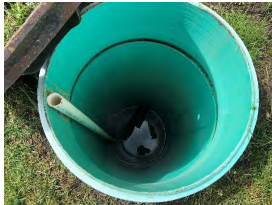
Figure 2-5 No Pump is Currently Installed Within the Sump Pit
