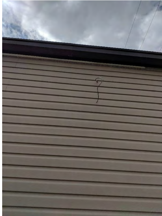
Figure 6-16 Exposed Wiring (North Side)
