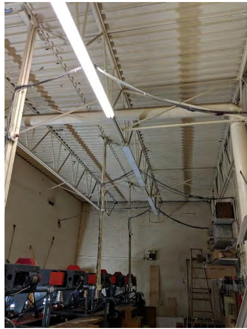
Figure 6-18 Service Aisle Room Lights Not Working
