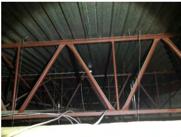
Figure 4-14 Viewing OWSJ Above Ceiling Space Above Bowling Lanes
