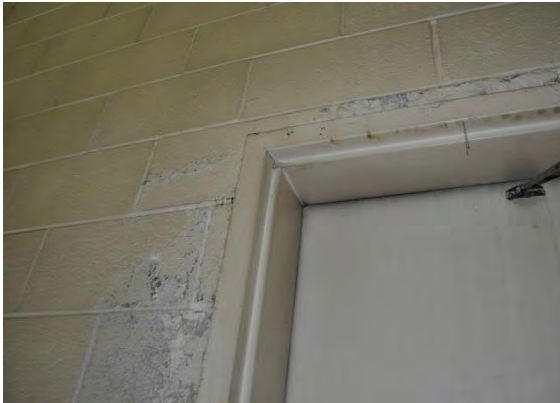
Figure 3-45 Water Infiltration Damage
