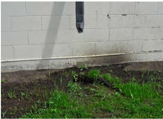
Figure 3-31 Downspout Extension Missing
