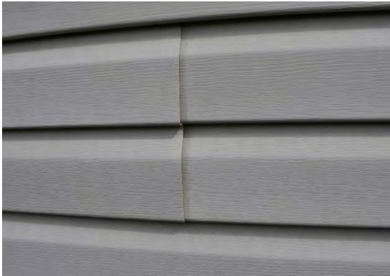
Figure 3-1 Signs of UV Deterioration
