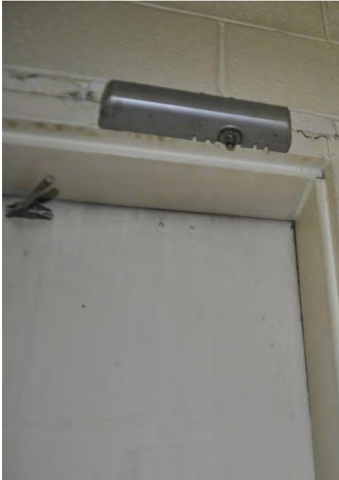
Figure 3-18 Door Closer and Water Staining
