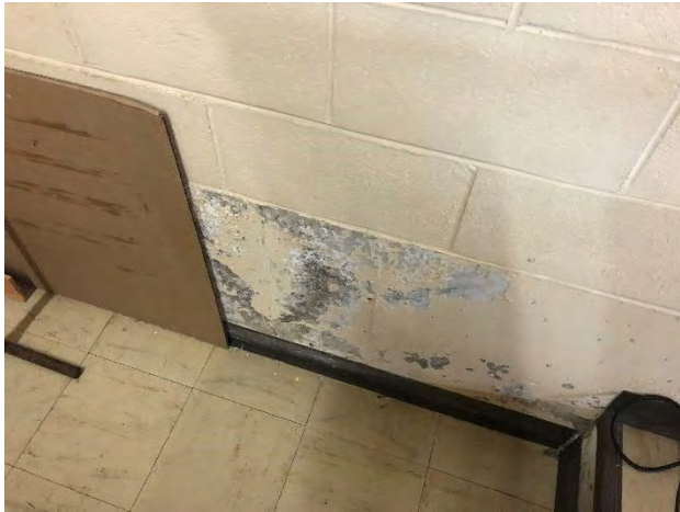
Figure 4-1 Efflorescence Damage of East Wall
