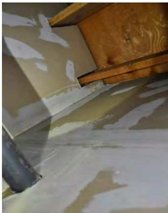
Figure 3-67 Mech Room Roof Joists (Not Fire Sealed)
