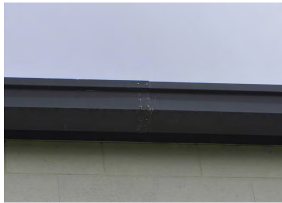
Figure 3-32 Gutter Connection
