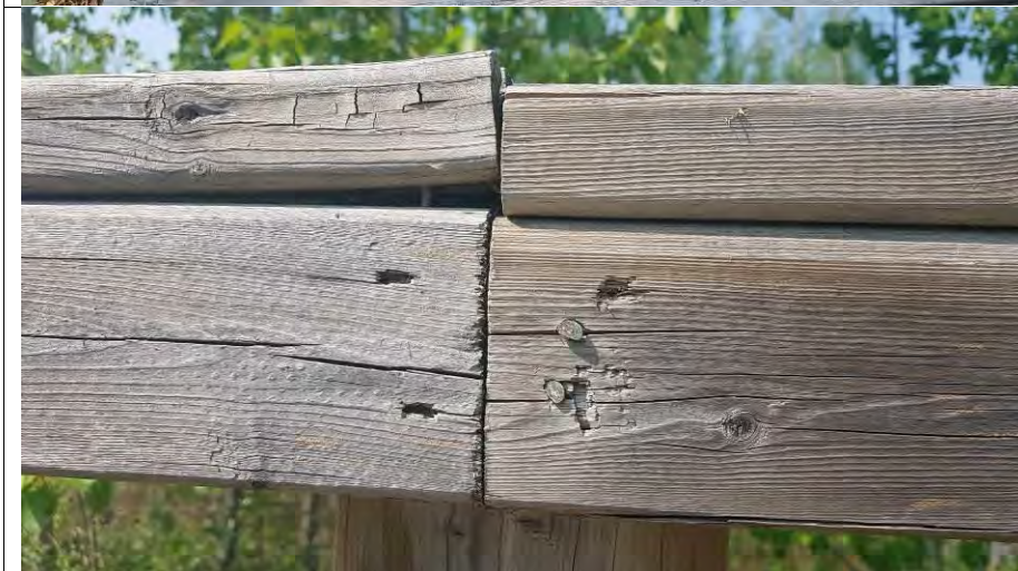
Photo 9 Loosening nail connections
