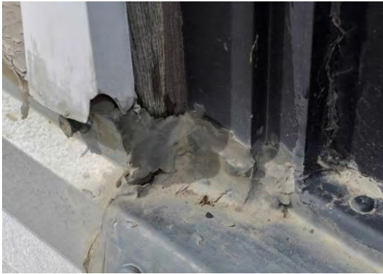
Figure 3-27 Clerestory Windows Flashing, Sealants and Cracking and Peeling Coating Over Glazing
