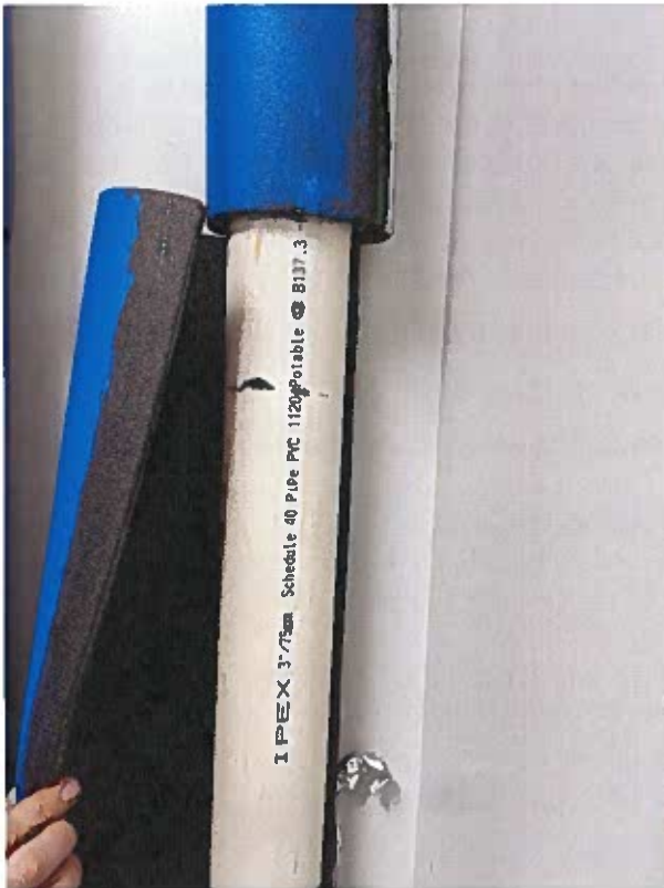
Figure 7 - Heat Pump Loop Piping
