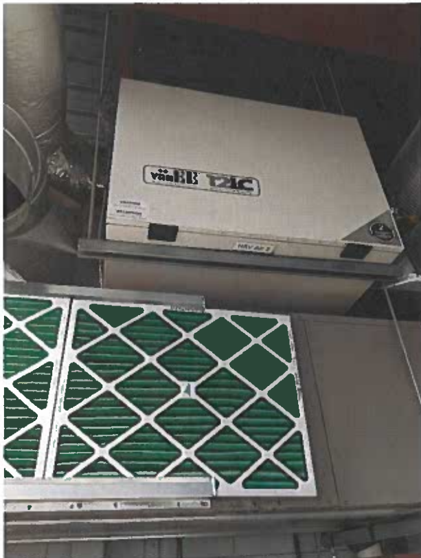
Figure 6 - Multi-Purpose Room Heat Pump and HRV
