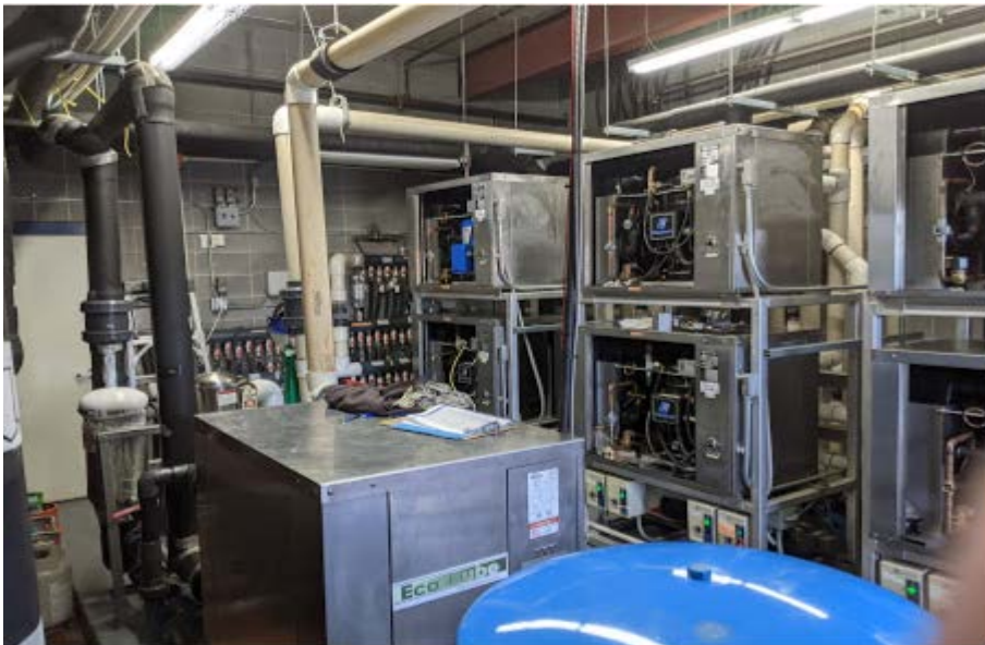
Picture # 1 – remove and replace the seven refrigeration pumps
