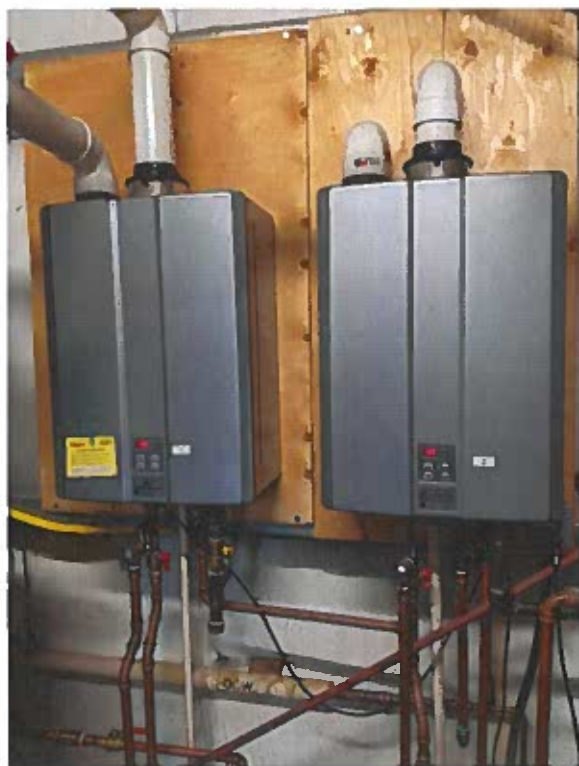
Figure 9 - On Demand Hot Water Heaters
