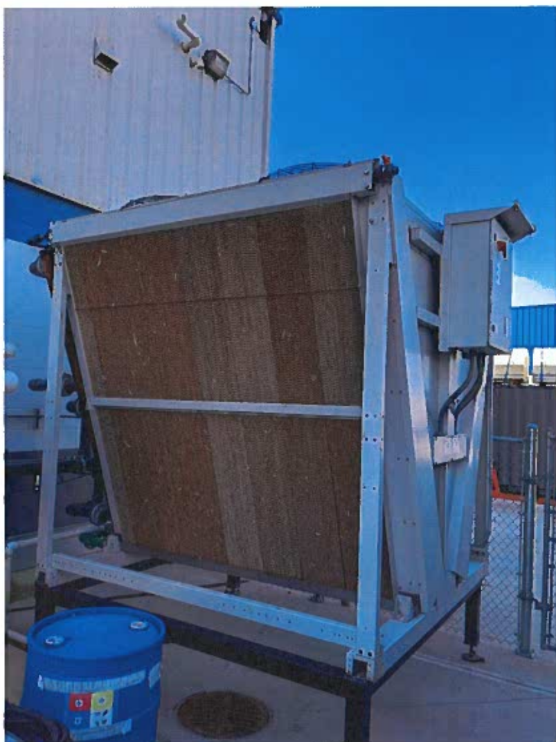
Figure 2 - Fluid Cooler
