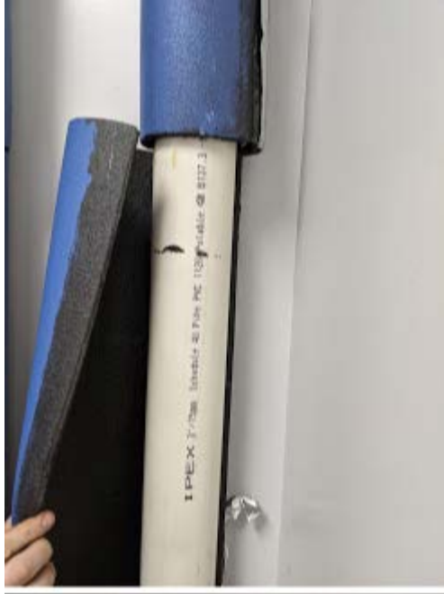
Picture # 2 – remove and replace approx.1,000 feet of heat pipe (some piping is warped)
