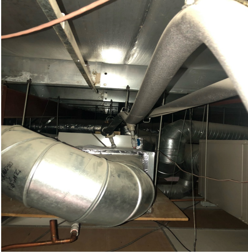
Picture # 3 - evidence of warped heat pipes
