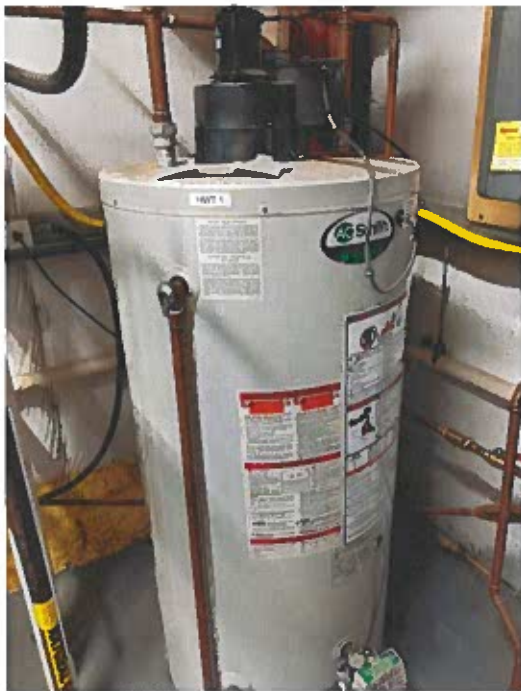
Figure 8 - Typical DHW Tank
